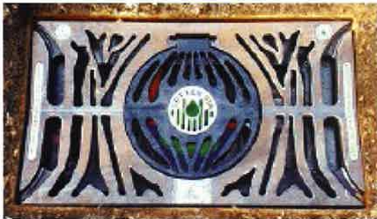
Top view of a Gutter Bin, Mundus Bag below grate capturing litter. Photo: Frog Creek Partners, LLC
