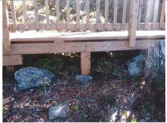
Photo 8. Showing post supports for ramp.
