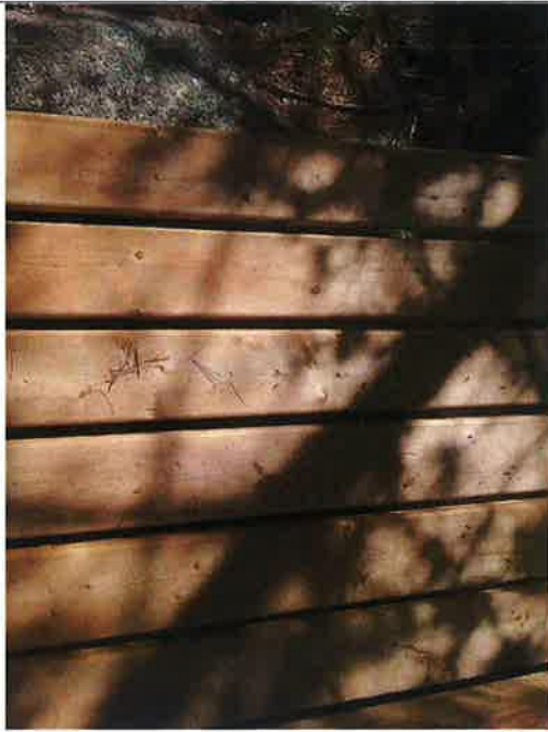
Photo 9. Board spacing on ramp
